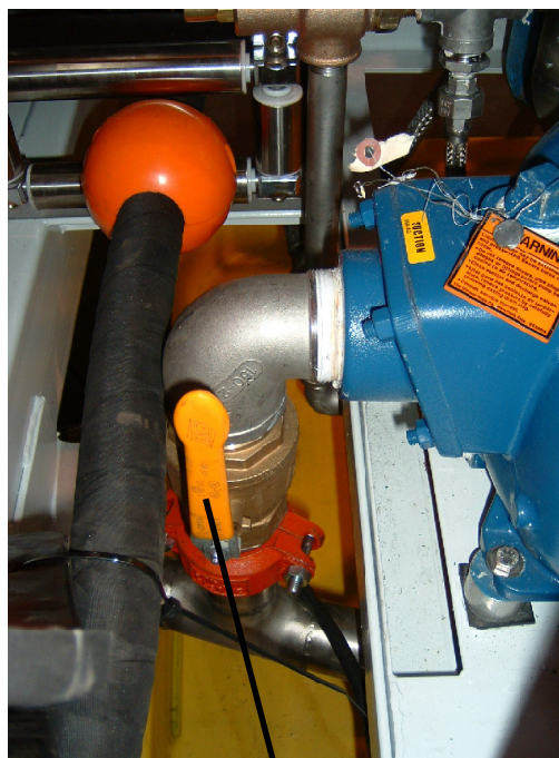
Fig 6.16 Pump Suction Valve on Inlet Side of Pump
